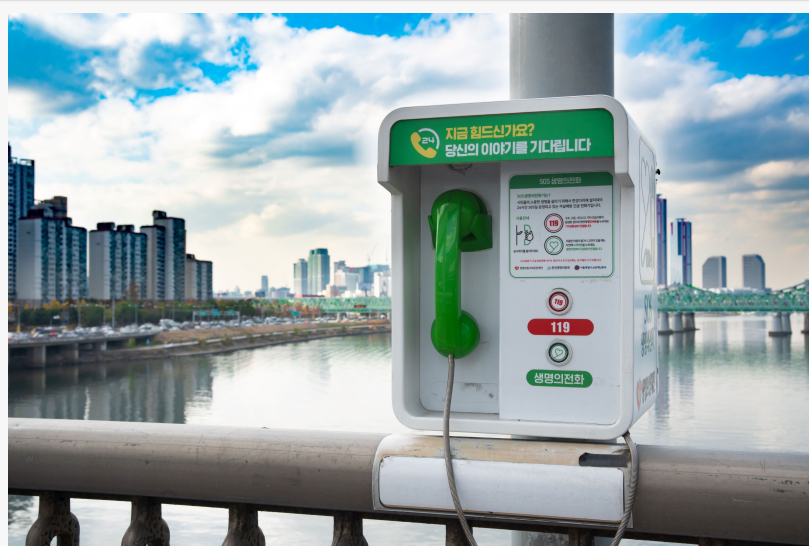
Emergency Phone on a Bridge
