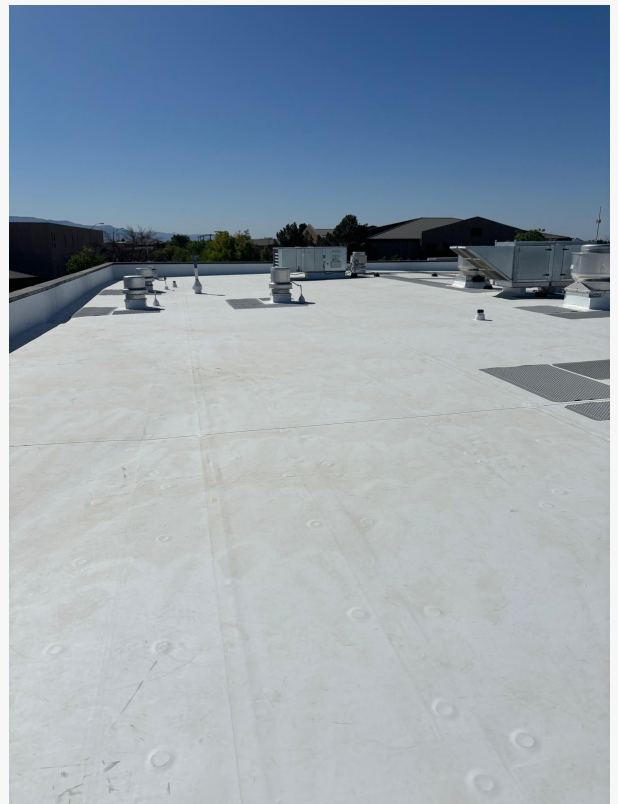
TPO commercial roof
