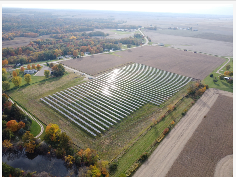
A Summit Ridge Energy 2.9 MW solar project located in Sparland, IL.
