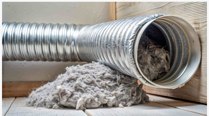
One of the most overlooked fire hazards in the home is the dryer vent.
