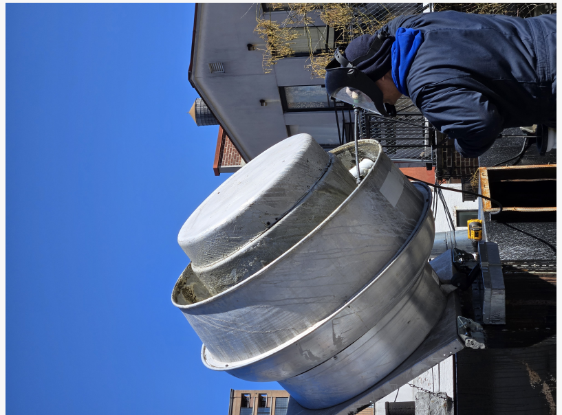
Hood Cleaning Technician Cleaning a Commercial Exhaust System in South Florida
