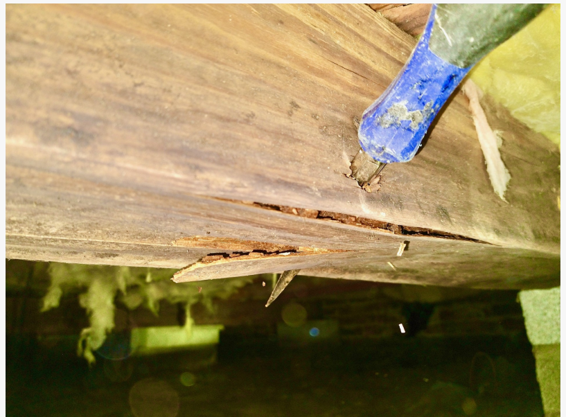
Brown Rot Damage to Floor Joist
