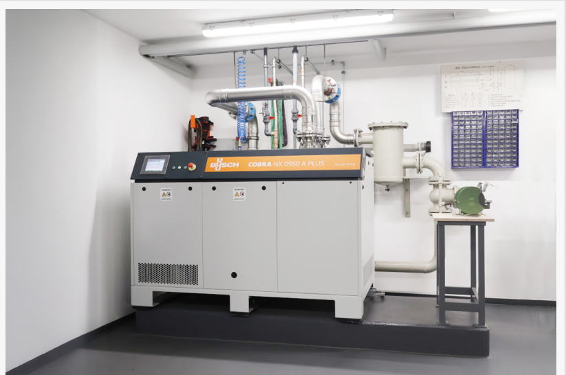
The COBRA NX screw vacuum pump provides reliable and efficient testing conditions. Source: Busch Vacuum Solutions.
