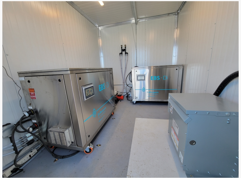
Installation of EBS-Di System in a specially designed trailer enclosure at the plant
