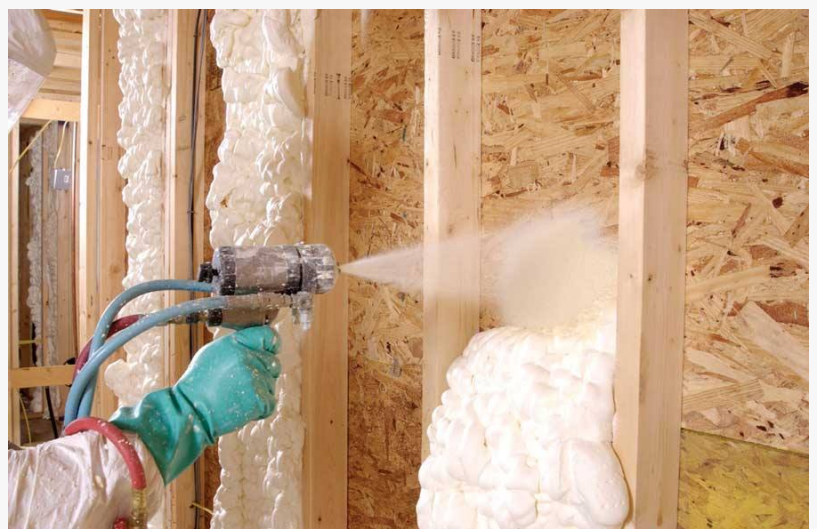
Spray Foam Insulation Process
