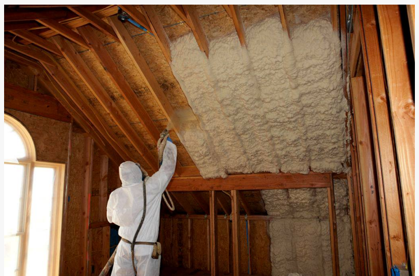
Professional Spray Foam Insulation Services
