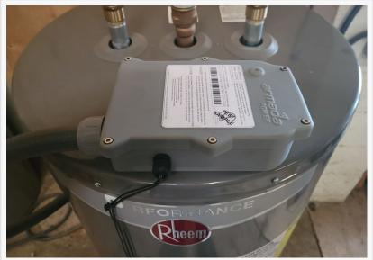
Armada Power's outdoor controller features a NEMA 4X waterproof design that allows it to be placed outdoors with no performance degradation.
