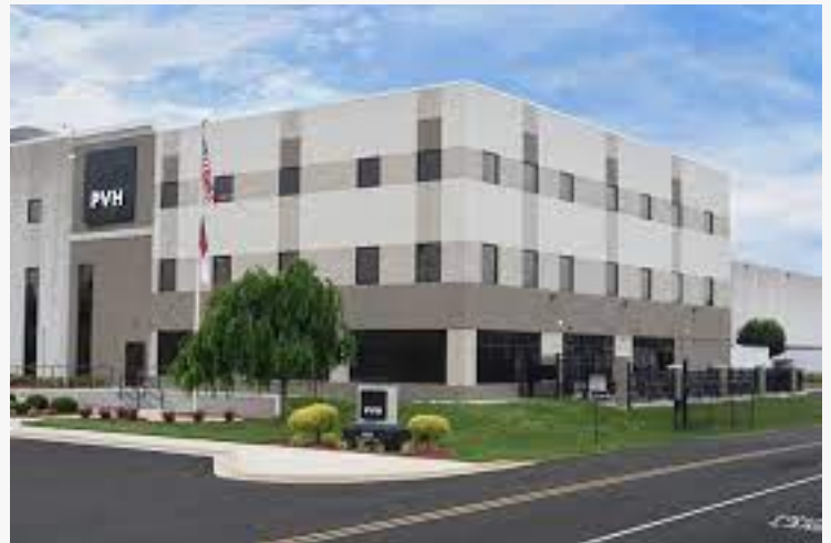
750,000 Sq. Ft. PVH Corporation Distribution Facility In USA
