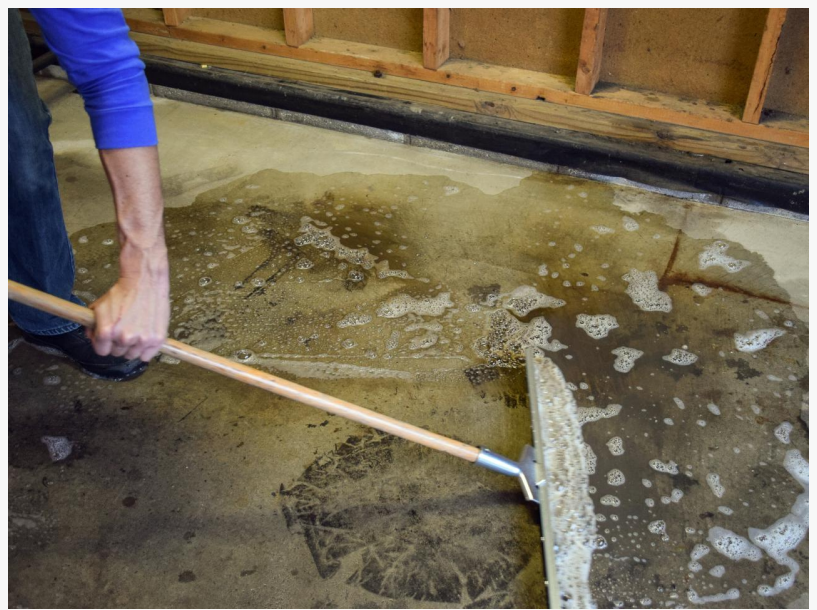
sweeping out sewage from garage
