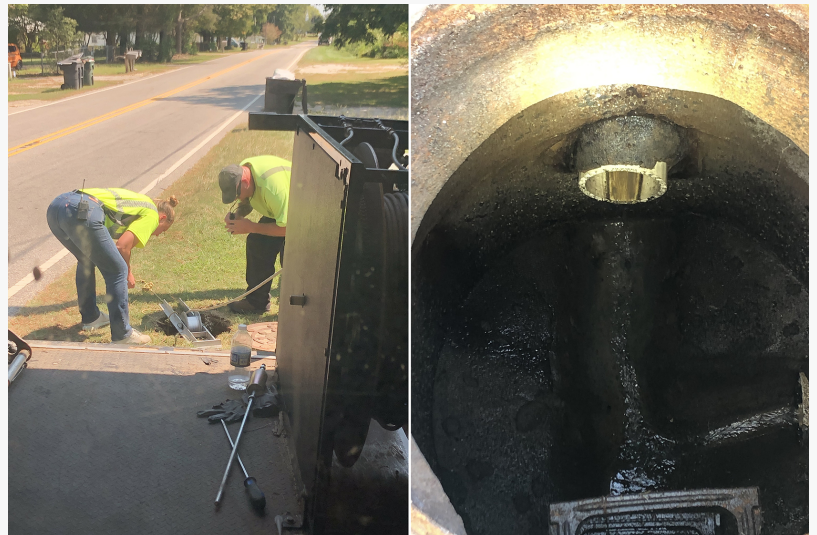
Electro Scan field workers positioning its intelligent probe to assess sewer pipes.
