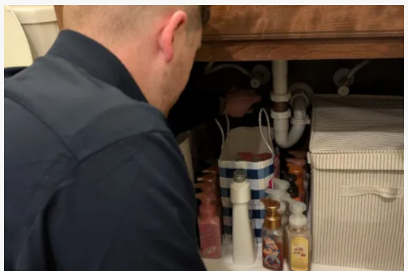
Mother Modern Plumbing offers $299 flat rate drain cleaning in Plano, TX.
