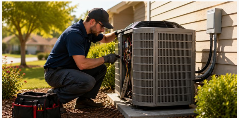
HVAC Technician Checking an AC Unit
