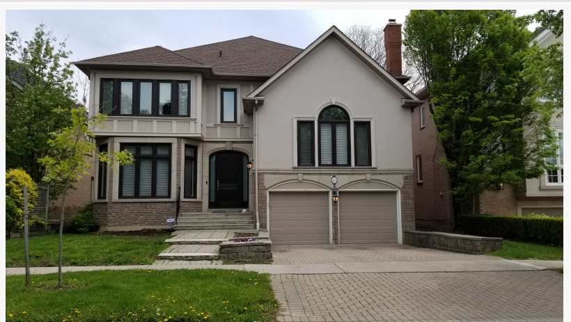
Full house windows and doors replacement
