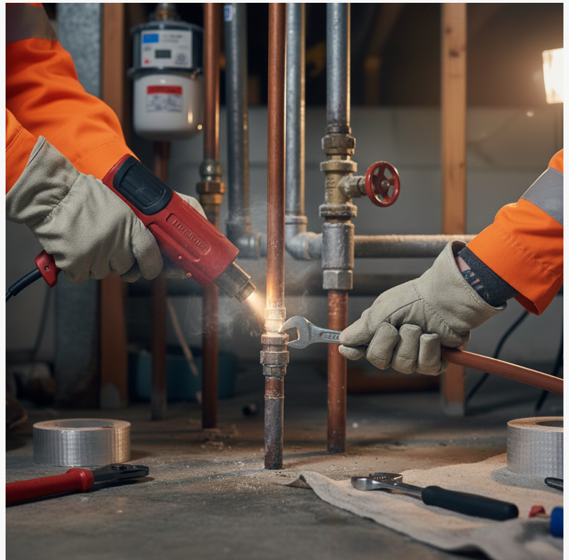
Plumbers heating and tightening copper pipe fittings during repair.
