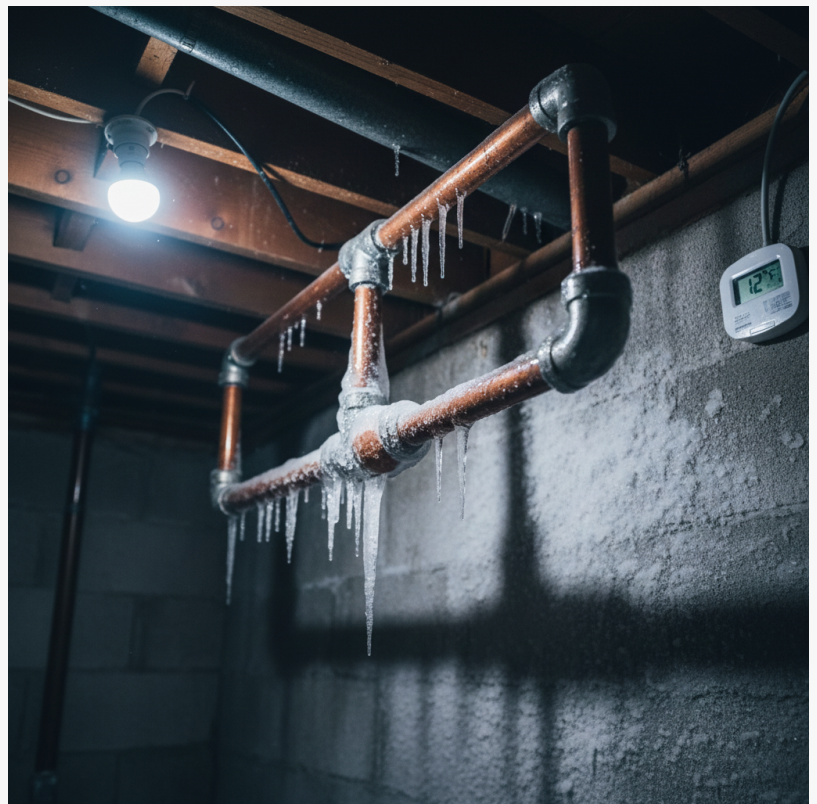
Frozen basement pipes covered in ice and icicles during extreme cold.
