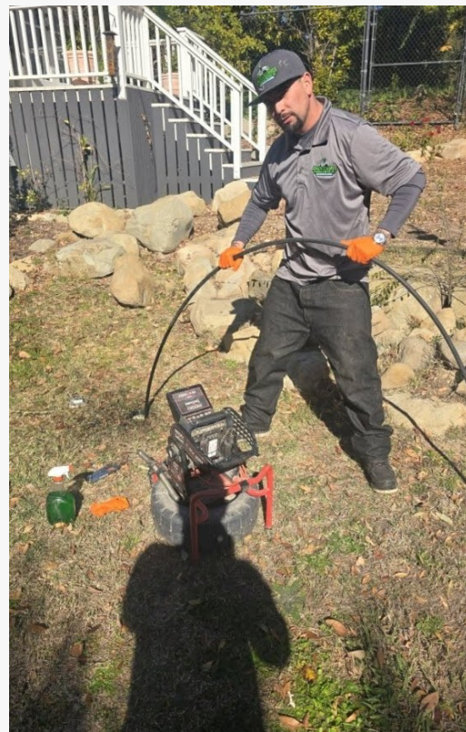
Hydo jetting drain cleaning with drain charmer plumbing & rooter, inc
